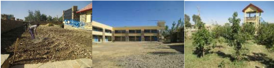
The new staff toilets (top right) behind The new classroom block The guard hut overlooks one gate and the gardens
